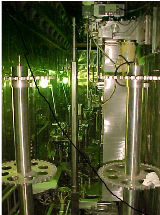
Machine to fabricate fuel assemblies
